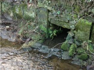
If you turn round and look downstream you will see the road bridge into Church Field. Down to the right is the opening of an old land drain. There are many drains bringing surface water into the beck at different places through the village. This is one of the older ones. Surface water running off the streets is far from clean. Such runoff is one of the main reasons Town Beck is in an ecologically poor condition.
