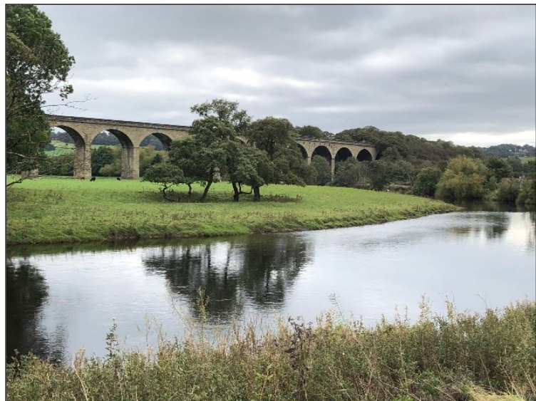
Zone 4: Arthington Viaduct
