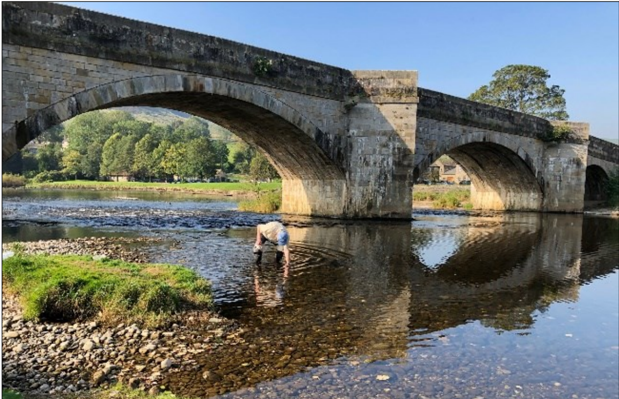
Zone 2: Burnsall Bridge
