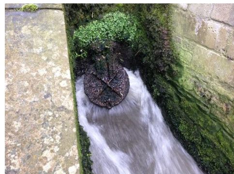
Figure 2: Treated effluent outfall
